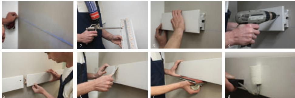
1. Make marks on surface of a wall with a level and chalkline to mount the cornice.
