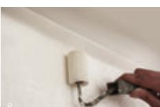
1. Prepare a hole in gypsum plasterboard that fits to a selected mounting element
