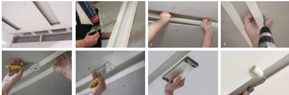
1. Prepare a hole in gypsum plasterboard that fits to a selected mounting element. The hole width shall match the size of the cornice without mounting lugs of the ceiling cornice
